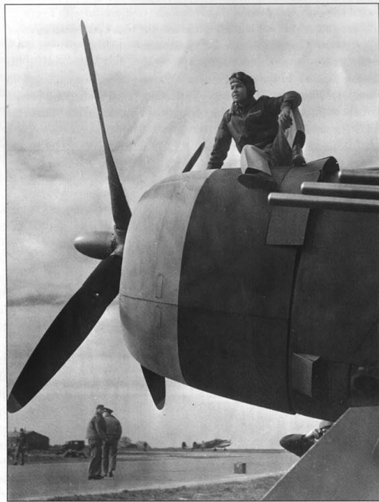
Press Day for the Thunderbolt, King's Cliffe, 10 March 1942. Lt Robert Stultz of the 62nd FS poses for size contrast on the cowling of P-47C 41-6209. The Pratt & Whitney R-2800 Double Wasp it housed was one of the most powerful, and hardy, radial engines ever built. This P-47, coded LM-V, was shot down on 30 July 1943, while Stultz fell victim to the Luftwaffe on 17 August that same year
